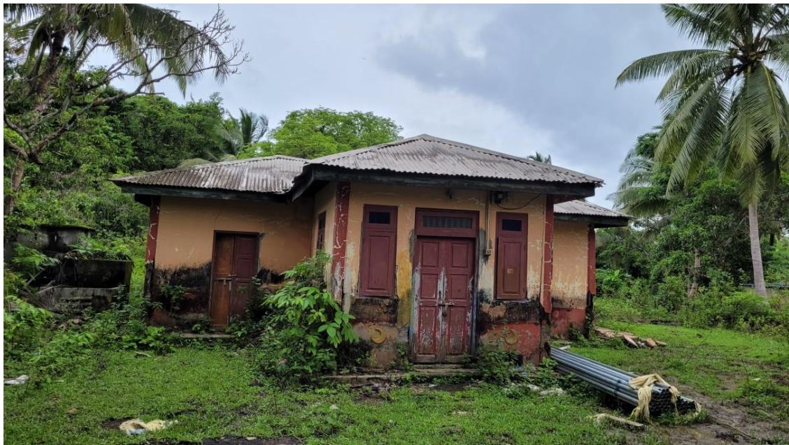
Photograph 11. An abandoned house that was severely damaged in the catastrophic tsunami in 2004 has become a haunting reminder of the destructive power of nature.
