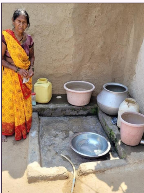
Photo 17: Water collected in buckets and utensils from a household pipeline connection under JJM
