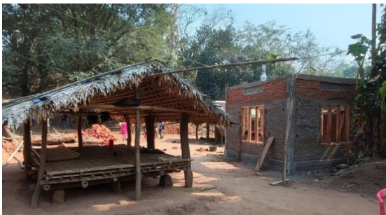
Traditional House and construction of P-MAY house
