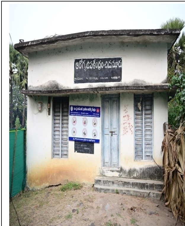
Fig. Anx.3.5. A Primary Health Centre in the village Chidumuru, Chintoor block of Andhra Pradesh
