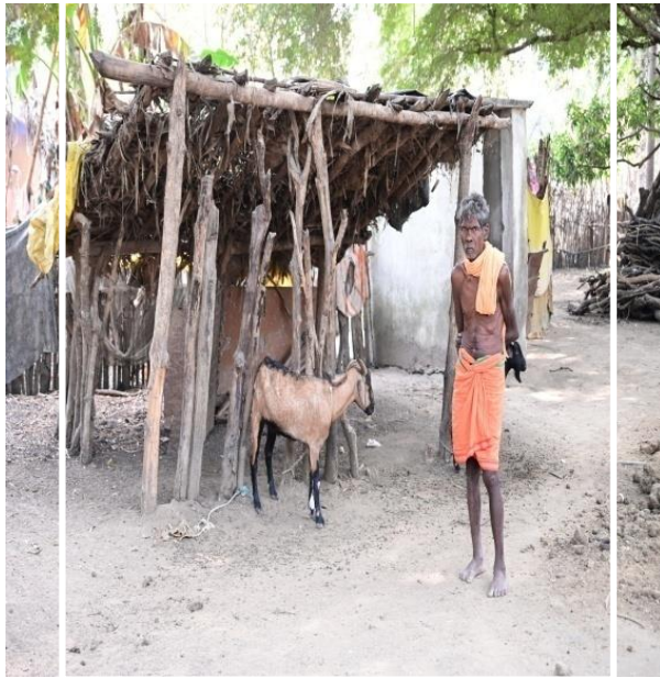
Fig. Anx.3.11. A goat shelter that is built in the ground level fashion
