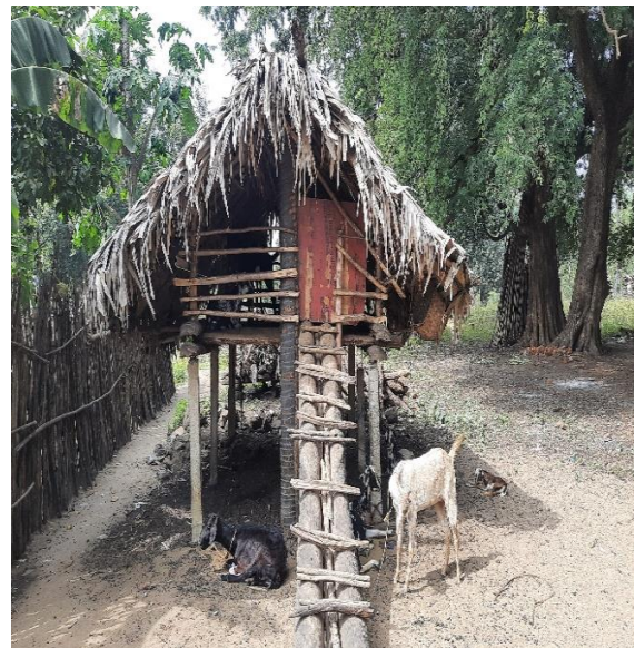
Fig. Anx.3.14. A typical goat shelter built above the ground
